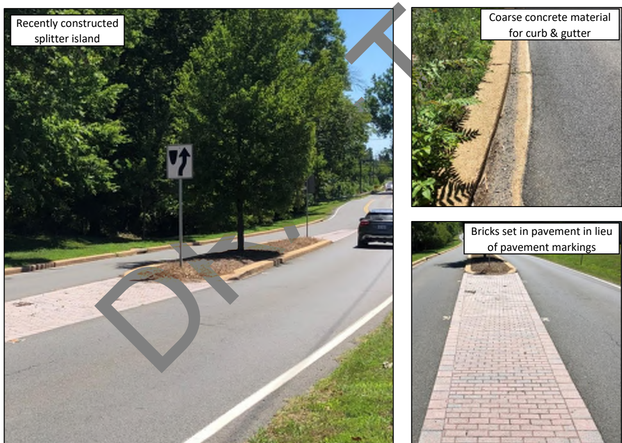
Figure 21: Pictures of Splitter Islands Constructed on Route 50 with Premium Materials
