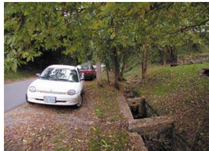
Antiquated Culvert along Water Street
