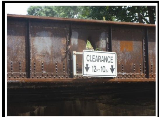
Figure 5.14. There are advantages for posting vertical clearance signs in advance of the obstruction. They can prevent overhead bridges that contribute to historic districts from being physically damaged by oversized vehicles. It does little good to place warning signs after the overhead obstruction has been hit. Photograph M. McCahon
