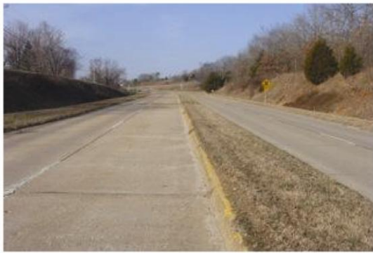
Figure 5.11. A concrete apron set into the integral curb on the concrete roadway is a historic treatment that appears to continue to function well given the condition of the bypassed section of US 66 in Missouri. Modern curbs and drop inlets would change the historic significance of the geometric design of the 1943 dualized highway. Photographs M. McCahon.
