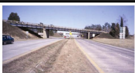
Figure 4.7. Historic Roads Need to Have Integrity As Well As Significance. I-85 Business at Lexington, North Carolina, built in the early 1950s, was one of that state's earliest limited-access freeways and was subsequently taken into the interstate highway system. An assessment of its integrity was critical to understanding the road as a historic structure and the refinements in roadway geometry that made it a "superhighway" in its time. The interchanges were considered so novel in this rural state that the department issued instructions to drivers about how to use exit and entrance ramps. This photo illustrates the median and shoulder treatments that were features of the original design. The roadway has significance within the statewide context of post-World War II urban bypasses. It remains largely as originally designed and meets the aspects of integrity. Photograph J.P. Harshbarger
