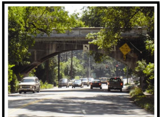
Figure 5.15. There are a handful of approaches to improving vertical clearance, including advance and on-structure signing and pavement marking. Unrestricted height crossings of this rail line are nearby. The overhead bridge and the roadway are both contributing resources to a historic district. Oversized vehicles must move to the inside lane in order to avoid striking the bridge. Photograph M. McCahon.
