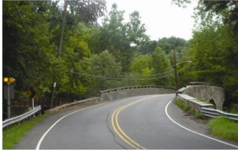
Figure 5.5. Signs can be used to warn in advance of sharp curves when there are constraints that preclude realignment, like on this early-19th century road with its stone arch bridge in a historic district near Princeton, NJ. Flashing chevrons and advisory signs were selected as the non-construction solution for several deficiencies, including alignments and superelevation. Note how striping has been used to mark and maintain travel lane width over the bridge while the shoulders are not. To accommodate pedestrians, the county placed a separate bridge (left of road bridge). All of these treatments preserve historic features while making the crossing as adequate as possible given the site limitations and strong desire by the community to retain the historic character of the district. Photo M. McCahon.
