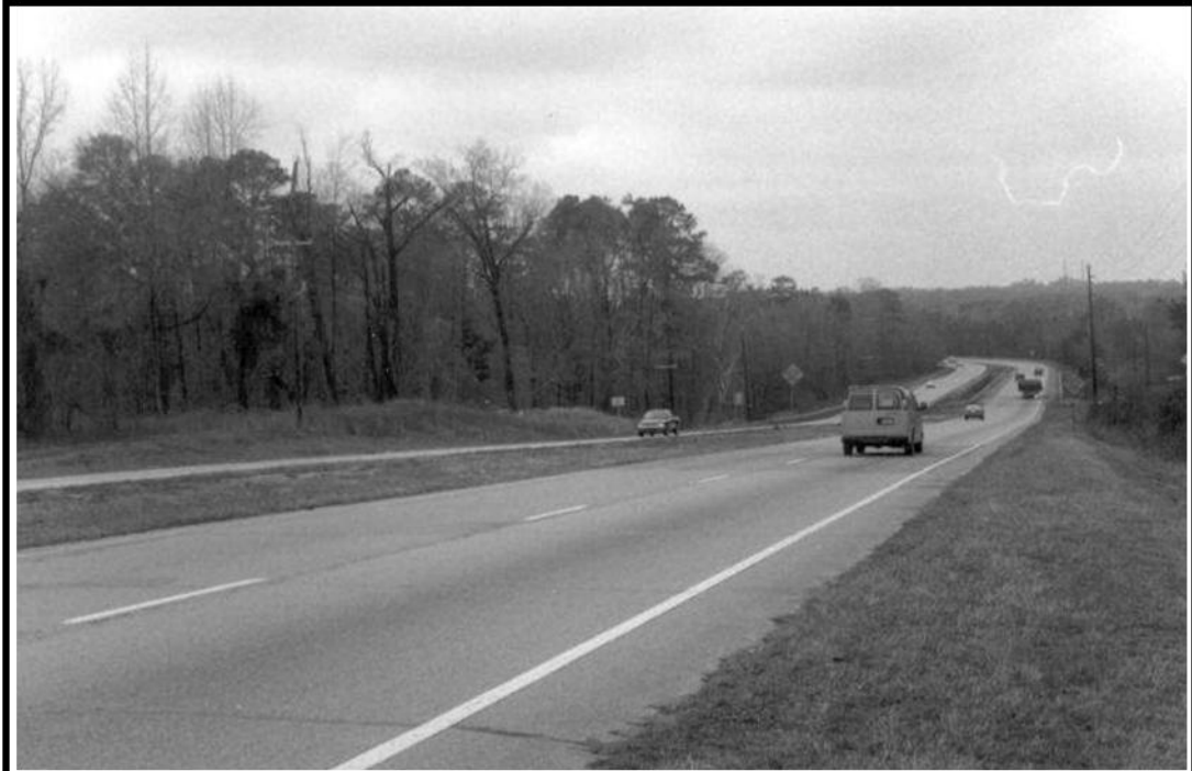
Figure 4.10. Historic Planned/Engineered Road US 27/Fort Benning Road (Georgia) Significance: First balanced-design road in Georgia applying federal-developed concepts, influenced all later designs and set standard that would be used over and over again on all later dualized (four-lane with median) highways (Criterion C). Significance established through statewide historic context for dualized highways. Integrity: Since balanced design is source of historical significance, location, design and association are the important aspects of integrity to consider. Significant features of road: design philosophy: design controls - speed, sight distance, grade, control of access all balanced in relationship to one another. Reflected in vertical and horizontal alignment, cross-sections, curve radii, use of a median, and construction of grade separation bridges located at points where military post roads could have access to the high-speed highway. Less significant features are the original pavement, shoulder treatments, side slopes, and railings.
