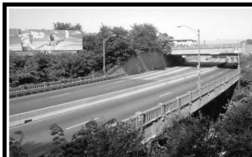
Figure 4.4. In response to the need to accommodate traffic approaching the 1923 Holland Tunnel through an already congested part of Jersey City, the New Jersey State Highway Department applied the economic theories of railroad location to a vehicular highway and built America's, and potentially the world's, first superhighway known historically as the Route One Extension. It is the quintessential engineered highway as it segregated through from local traffic and made provisions for changing grades along the limited-access, dualized highway that also passes through the Bergen Ridge as it approaches the at-grade tunnel portal. Most of its geometric features contribute to its historic significance. Because the highway was literally wedged into the existing fabric of Jersey City, the portion of the road from the tunnel to the south end of the Pulaski Skyway could not be widened. A completely new road on a new alignment (Jersey City Extension to the New Jersey Turnpike) was constructed in the 1950s to increase capacity. Its construction largely ensured that the historic road would retain its integrity. Photographer: Thomas Flagg.
