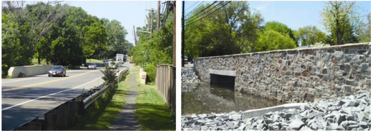
Figure 5.9. The crossing is located in overlapping historic districts, each with its own significance. The bridge was originally built in 1907 as part of a lake developed for rowing regattas, and as such it was an incident in a manipulated landscape as well as a transportation facility. The highway itself was listed in the National Register as an evolved highway dating to the colonial era. It was taken into the state highway system in 1919 and subsequently upgraded using AASHTO design criteria. The National Register nomination was prompted by local desire to limit truck traffic or increase in roadway width. Consequently, the unimproved pavement edge treatment is very important to local stakeholders, who also wanted the new bridge and clear zone to accommodate pedestrians. In order to not adversely affect either historic district, the new bridge was finished with stone-veneered fasciae. It continues to serve as a frontispiece in the lake-centric historic district. The pedestrian bridge was integrated into the roadway bridge, and the desired sidewalk was finished as stabilized earth so as to maintain the historical unimproved pavement edge treatment. The standard safety-shape barriers were finished with tinted concrete. The bridge is in a suburban setting dominated by post-World War II houses in Princeton New Jersey. Photographs M. McCahon.
