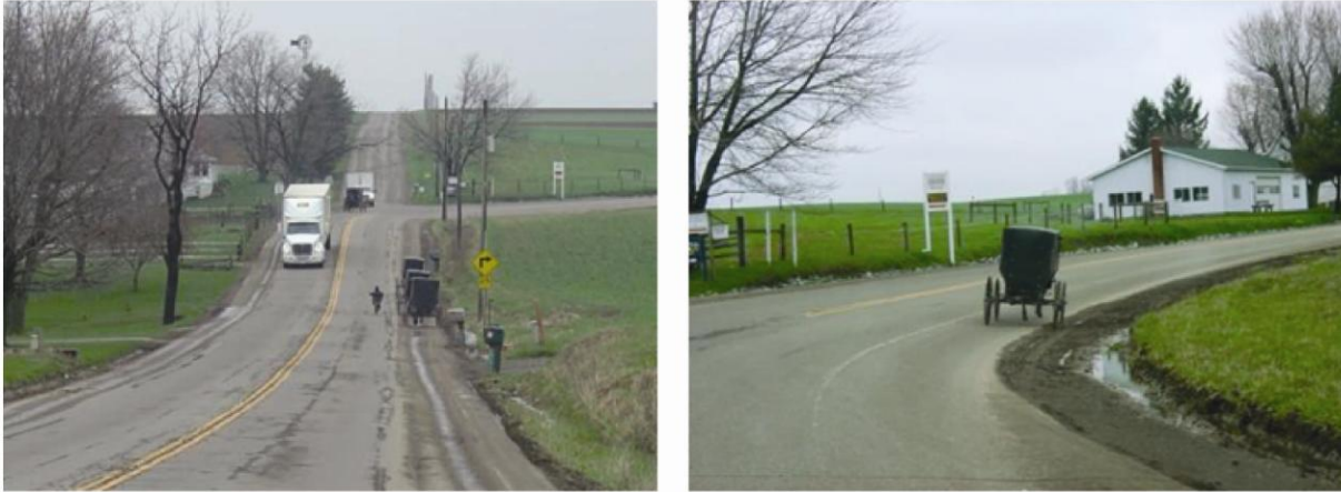
Figure 5.8. There is a wide range of flexibility for shoulders depending on local conditions. One of several treatments could be applied to increase the safety and operations of this segment of state highway for its multi-modal uses, including incremental widening of the travel lanes and shoulders, which in this locale also serve as a buggyway. Note that even the buggies off track on the inside of the curve. Enhanced pavement markings could improve the ability of motorized vehicles to stay in the appropriate travel ways, especially on the inside of the curve as buggies labor up the hill. Photographs M. McCahon.
