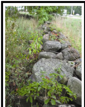
Figure 3.3. The dry laid rubble stone wall located near Chichester, NH was reconstructed in 1993 in accordance with the state DOT's administrative policy on rebuilding stone walls parallel to roadways. Photograph courtesy of Marc Laurin, NHDOT.
