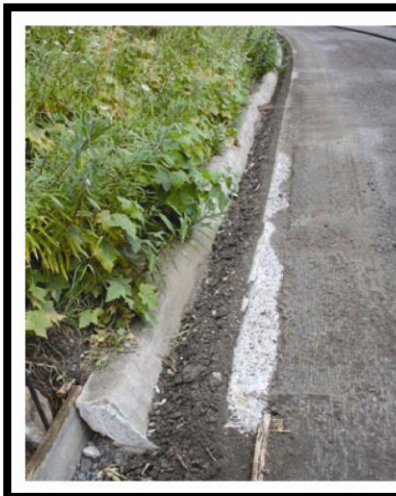
Figure 5.6. On the Historic Columbia River Highway, the removal of generations of asphaltic overlay brought back to the original Warrenite pavement (lighter color), an early 20th century proprietary bitulithic paving material. This has also allowed for the restoration of the concrete gutter system. Photo courtesy Robert Hadlow, Oregon DOT.
