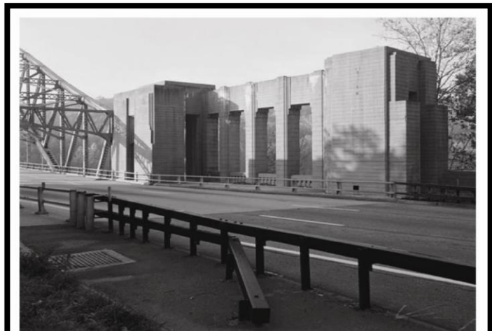
Figure 5.18. Barriers are an appropriate treatment to shield a historically significant object or fixture. Here barriers are placed between the roadway and the Art Deco-style pedestrian overlook at the Croton Reservoir Bridge on the Taconic State Parkway in New York.
