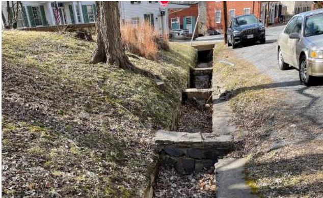
Existing concrete-lined channel along Water Street
